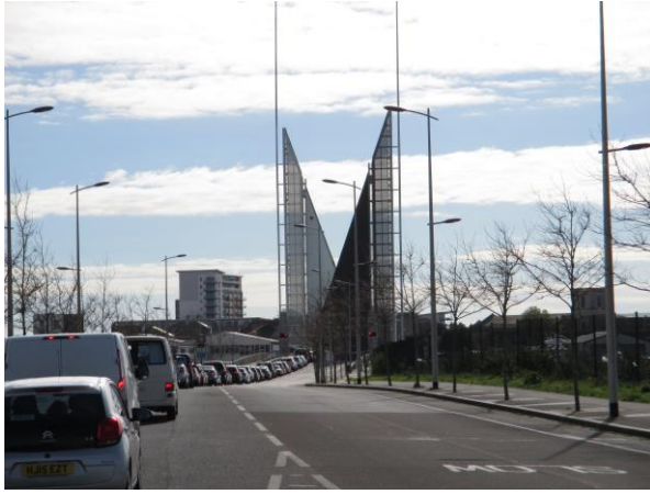
Twin Sails Bridge, Poole
