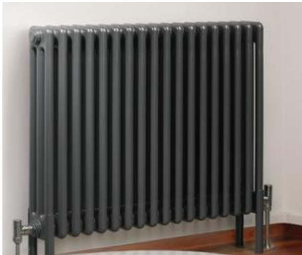
Tubular steel radiator suggested to replace the existing cast iron units. Alternative colours and valves are available.
