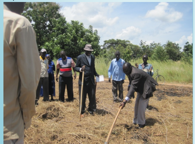
The Commissioner breaks the ground for the Health Center
