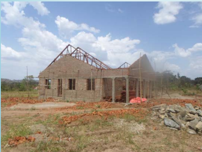
The construction status on 10 th March 2016
