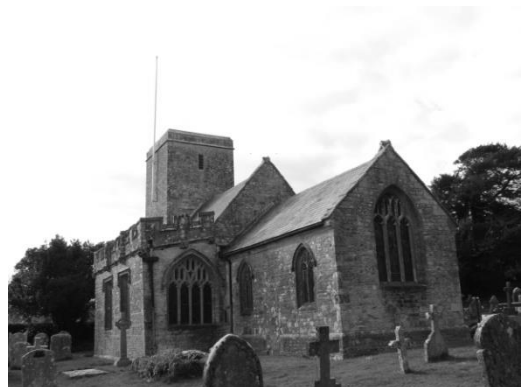
Stinsford Parish Church; PV panels are cleverly hidden behind the parapet.
