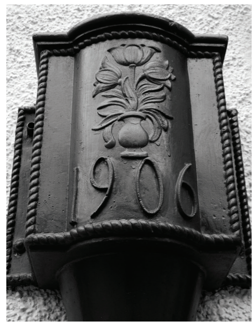
Thorpe Lodge drainpipe with its dahlia insignia
